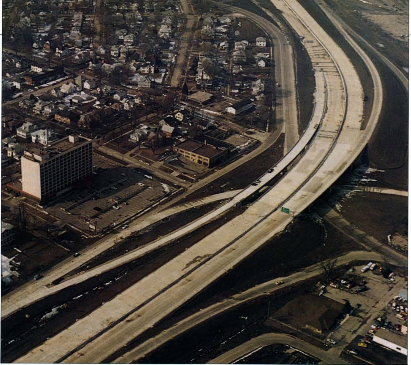
Cedar Valley Corp. is building Highway 218 through downtown Waterloo. The project is a six-lane divided highway with multi-lane service roads on each side. The $10.5 million, 1.5 mile first leg is scheduled to be completed this summer. Two other stretches by Cedar Valley Corp., amounting to $17 million, are scheduled for completion by fall.
